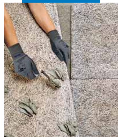
Laying heavy insulation panels
