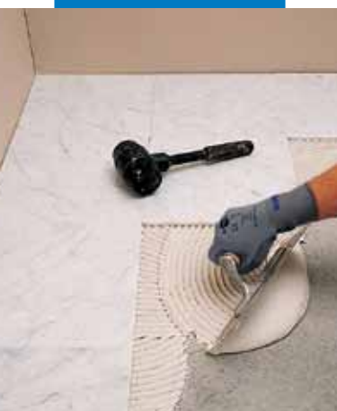
Setting white Carrara with Keraquick white
