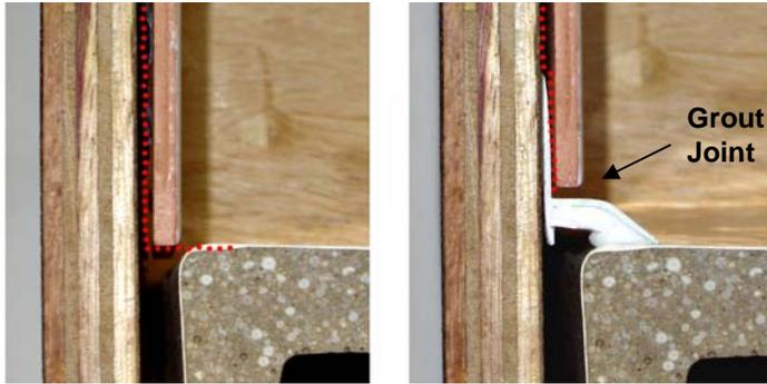
**Solution:** The installation of a British Standard compliant movement joint seal such as Sealux 20 can bridge wall/ledge gaps up to 12mm. This makes waterproofing possible over all shower trays and baths.
