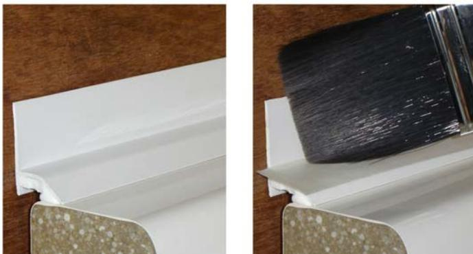
**Solution:** This task is made easier and quicker by first installing Sealux over the joint, masking the strip and dressing the membrane down over the up-stand.
