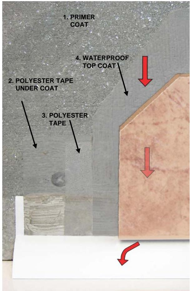
**Solution:** Install a Sealux movement joint seal. When tiling, grout the tile/strip joint. The grout remains bonded to the tile while the joint between the grout and strip acts as a *release line* that prevents the build up of moisture.
