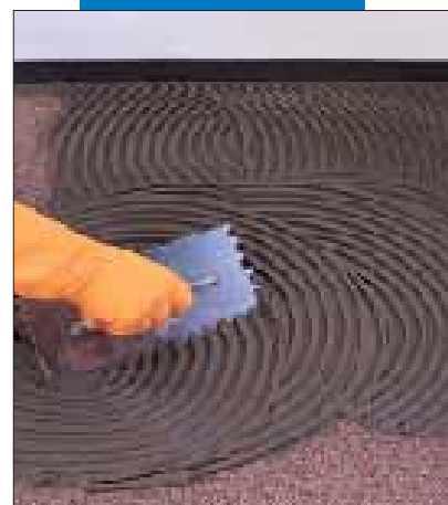
Applying the Mapeconic Mortar over the Mapeconic Pads
