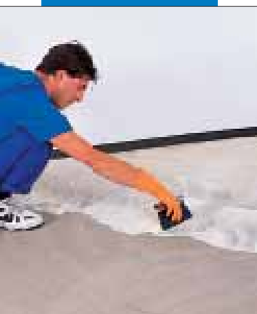
Applying Mapeconic Glue with a notched trowel
