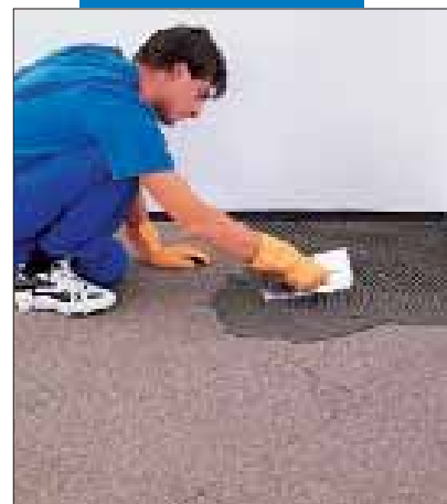
Applying the Mapeconic Pads
