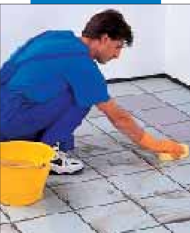
Cleaning the flooring with a damp sponge
