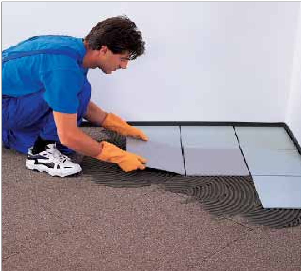
Installing polished porcelain tiles
