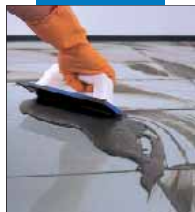
Filling joints with Mapefonic Grout
