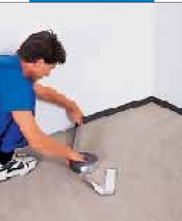
Applying Mapeconic Strip around the perimeter of the room
