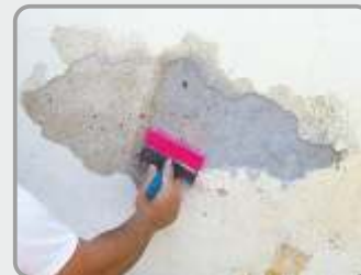
The surface is primed with FLEX-PRIMER or NANO-SEAL and the surface is stabilized.
