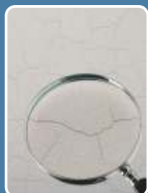
Extended cracks to plaster out of being an aesthetical problem, may sometimes also be dangerous for the plasters durability against water and freeze.
