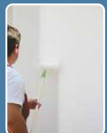
Two more layers of FLEXCOAT should be applied in order to cover the polyester fabric ( TREVIRA ). Without using TREVIRA only one more layer of FLEXCOAT is enough.
