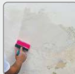
As soon as the plaster has dried, the surface is primed again with FLEX-PRIMER .
