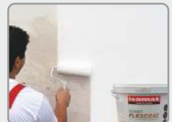
Finally, the surface is painted with two layers of FLEXCOAT .
