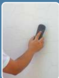
Substrate should be thoroughly cleaned from dust etc.
