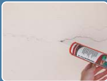
The crack is sealed with elasto-plastic acrylic sealant ISOMASTIC-A .
