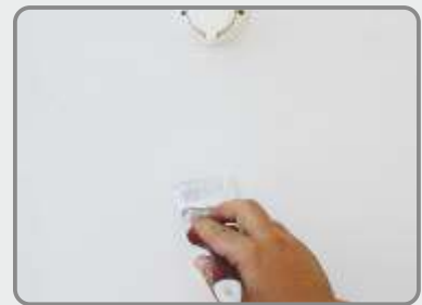
The 2 nd layer of FLEXCOAT is applied after the first one has completely dried.
