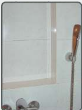
Moisture problems to rooms adjacent to bathrooms or kitchens appear because the tile grouts are absorptive.
