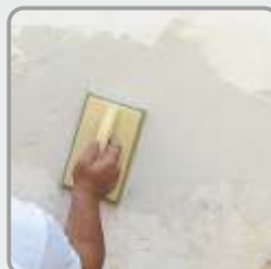
After the plaster has been sufficiently set, it is smoothed by hand with a spongy float.
