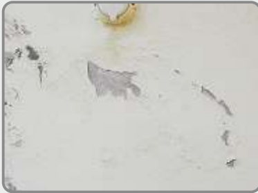
Damaged colour is the first indication that the plaster is corrupted from water.
