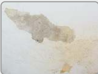
Crumbling plasters are a common phenomenon for walls with moisture problems.
