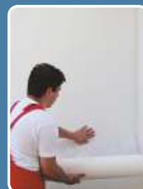
In cases of multiple cracks, the first layer of FLEXCOAT is reinforced, while it is still fresh, with the polyester fabric ( TREVIRA , 100 cm width).
