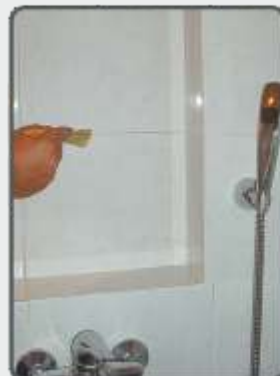
NANOPRO-C is applied with brush along the joints in two layers.
