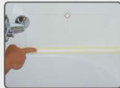
The sealant is formed while it is still fresh.
