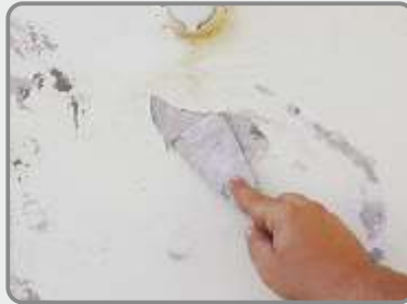
Old colour should be scratched with a spatula and the loose particles should be removed.
