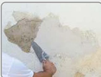
The plaster is fixed with the repairing mortar UNICRET-FAST , improved with the resin ADIPLAST .
