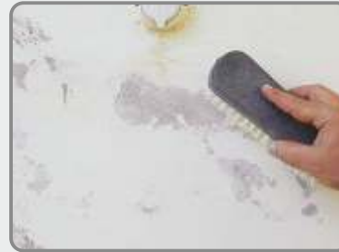
Substrate should be thoroughly cleaned from dust etc.
