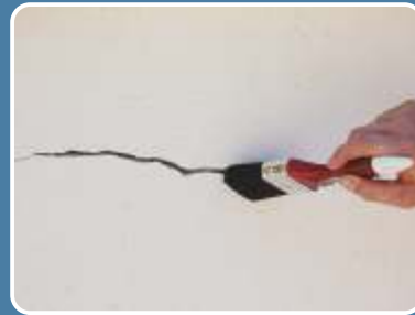
Crack should be thoroughly cleaned from dust.
