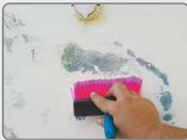
The surface is primed with FLEX-PRIMER .
