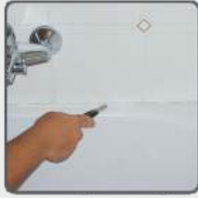
The old sealant is removed mechanically (by chisel etc.), trying not to damage the sanitary ware. Then the surface is cleaned with alcohol.
