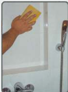
The tiles are cleaned by using a wet sponge.
