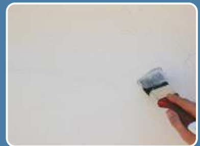
After ISOMASTIC-A has dried, the crack is painted with FLEXCOAT along its length.
