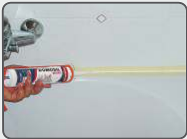
The intersection is sealed with the mildew-resistant silicone sealant DOMOSIL-S or DOMOSIL-MICRO .
