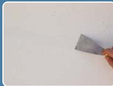
While the sealant is fresh it is formed with a spatula.
