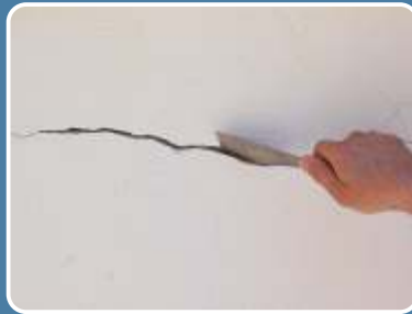
Wherever it is required, the crack is opened with a spatula in a width of 3 mm.
